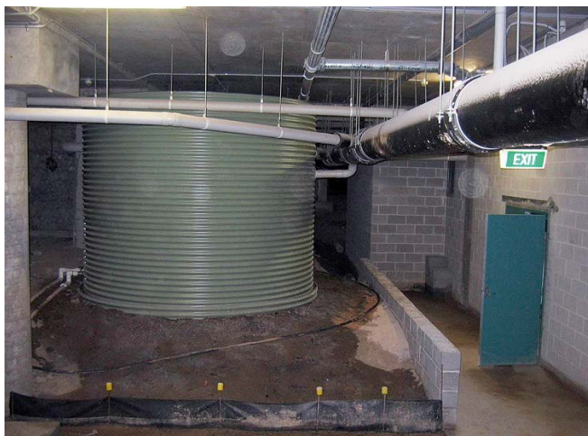
Example of a basement intercept “without overflow”
