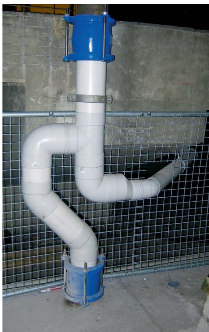
Example of a peak flow diversion
